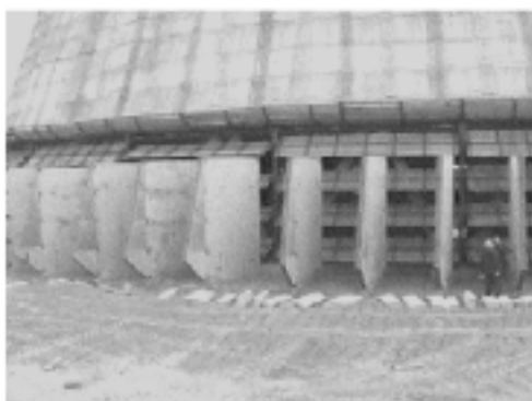
Fig. 10. Production prototype of an aerodynamic vortex generator.
